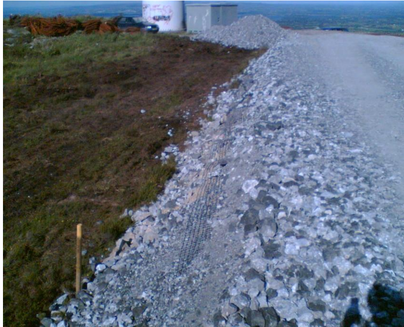
Figure 4-7: Illustration of suitable road surface and drainage
